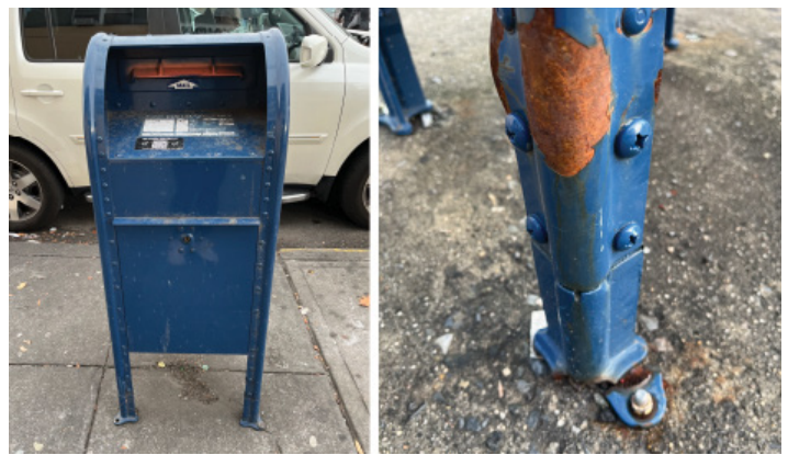
Figure 4. Queens, NY Blue Collection Box With Missing Bolts and Corrosion
