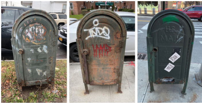
Figure 5. Queens, NY Green Relay Boxes With Door Gap, Missing Bolts, Cracks, and Corrosion
