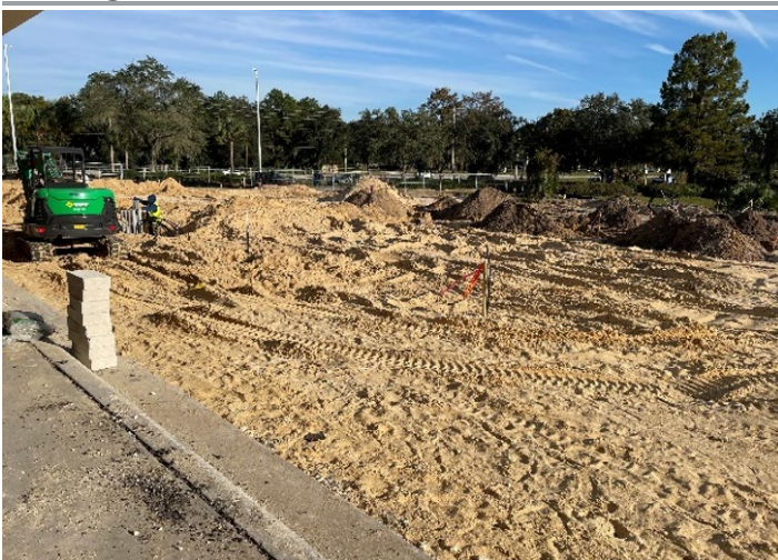
Figure 4. Construction at Gainesville S&DC Parking Lot
